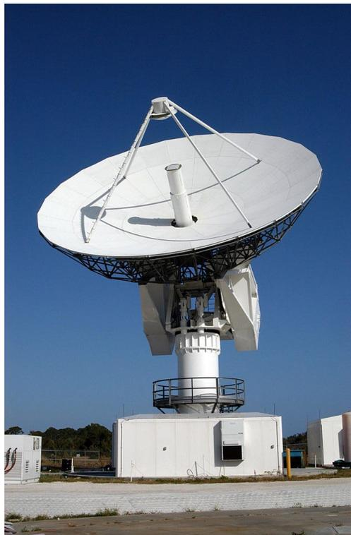
**Figure 5. Radar Paraboloid U.S. Army C-Band Radar Dish Antenna [6].**
