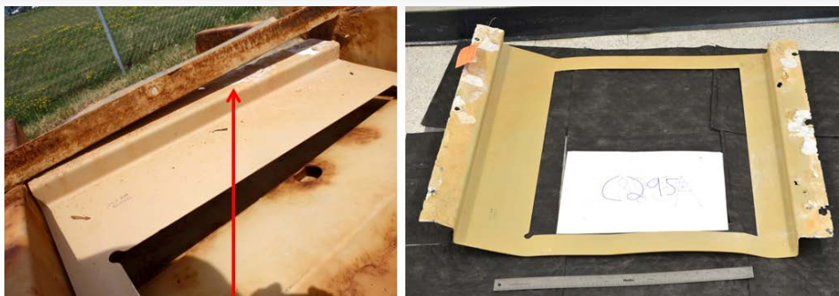
Figure 8: Transmission Cooling Shroud Crevice and Galvanic Corrosion at Bolted Joints and Water Entrapment Area [2].
